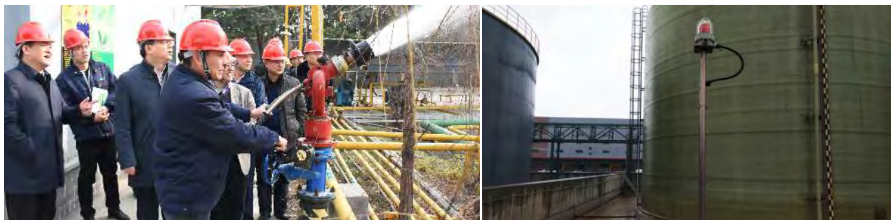
Liquid Level Alarm of Fire Water Gun
